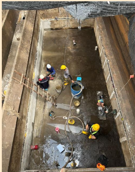
Existing Filter No.4 - Refurbishment work
