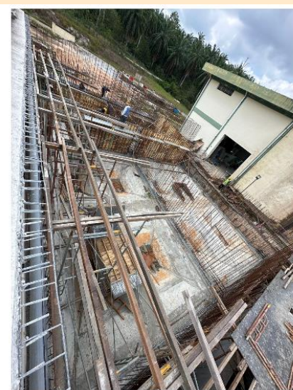
New Sedimentation Tank 2&3 - Reinforcement and formwork work
