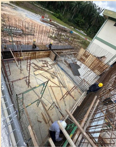
New Flocculation Tank 2&3 - Reinforcement and formwork work
